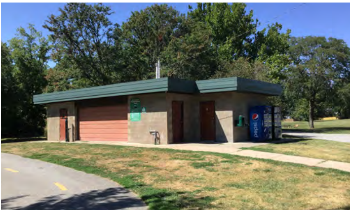
Restroom and Storage Facility
