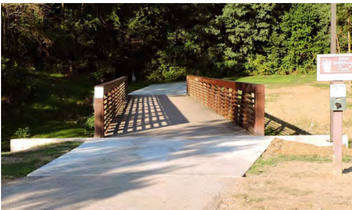
Bridge Improvements - Summer '21
