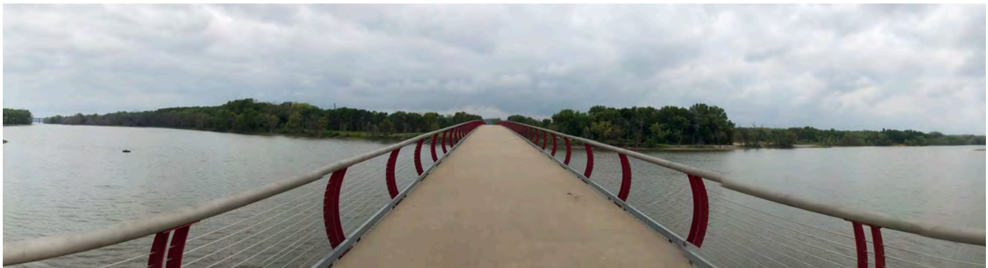
Panoramic of Pedestrian Bridge
