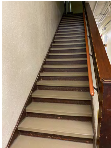
Staircase to Second Level
