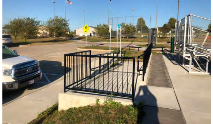
ADA Ramp to Miracle Field
