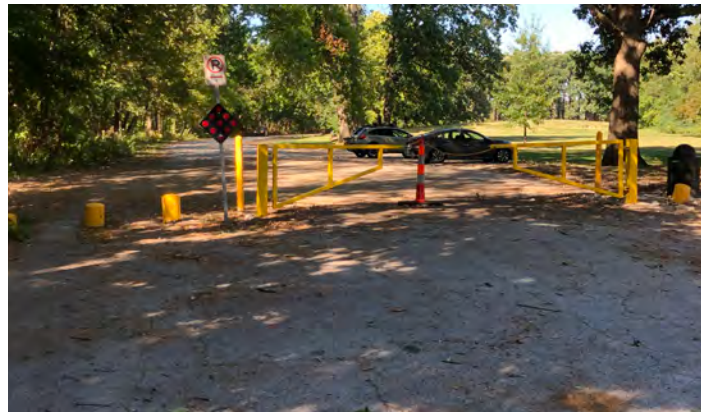
Traffic Control Gate near Tennis Courts
