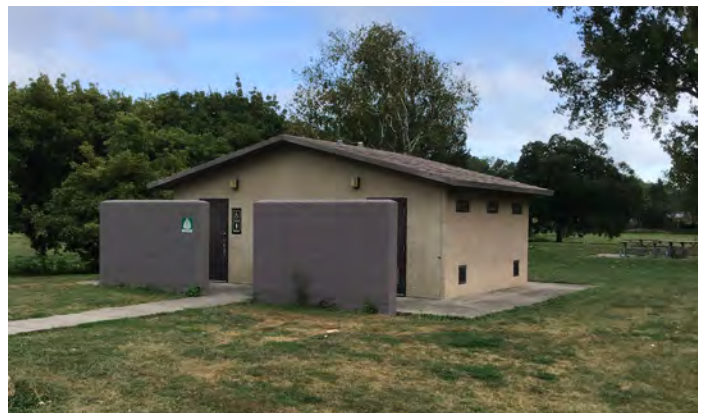
Restroom Facility PARKS CONDITION ASSESSMENT
