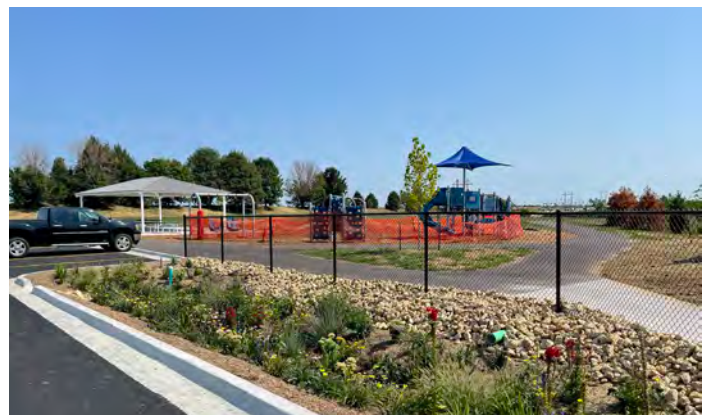
Bio-Swale with Playground in Background
