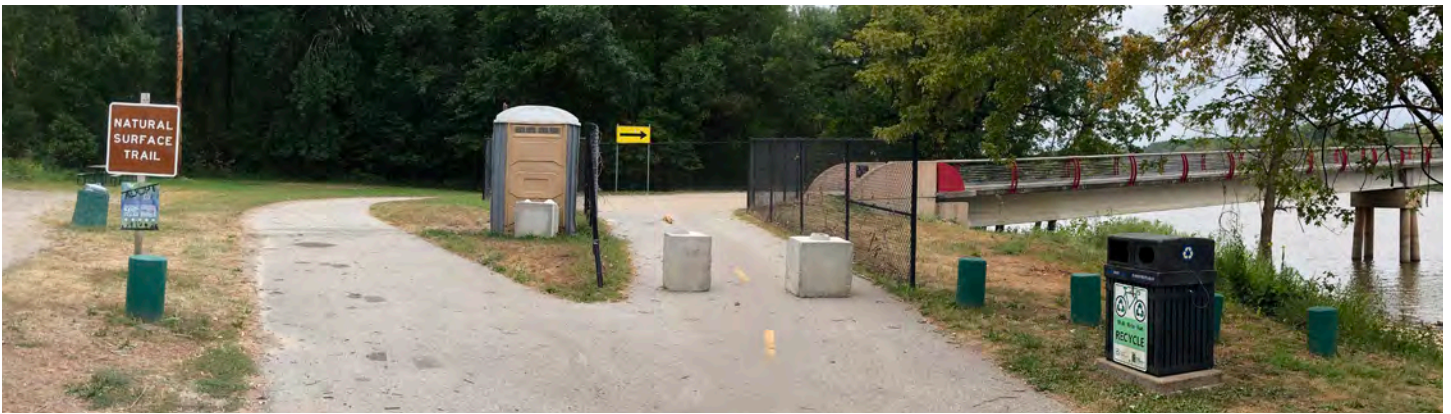
Pedestrian Bridge Access from Credit Island
