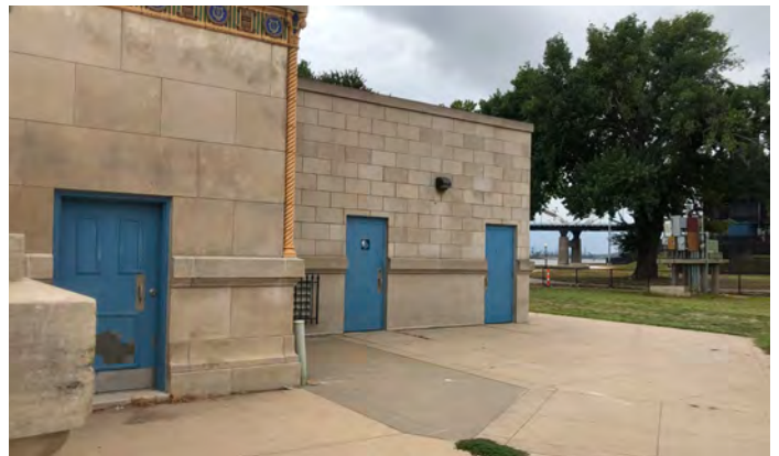
Restroom and Storage Facilities
