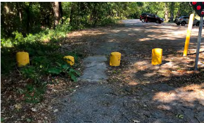
Pedestrian / Cycle Access Through Gate
