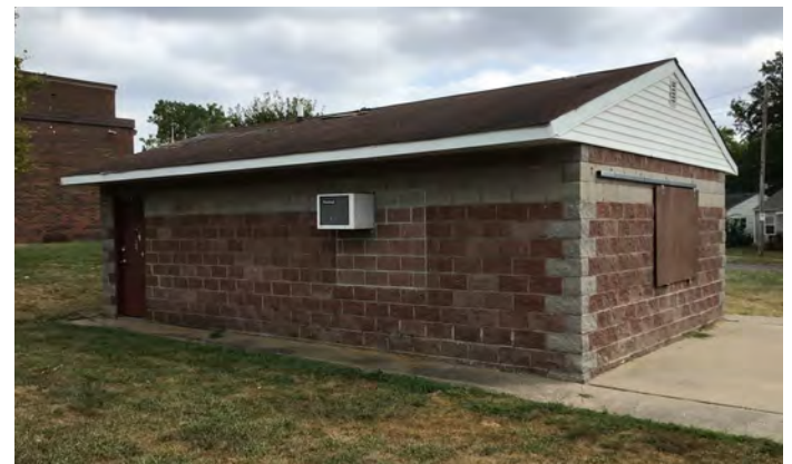
Concessions and Restroom Facility
