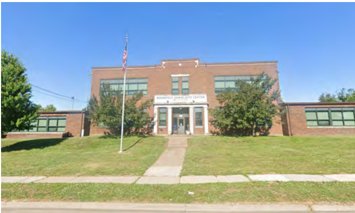
Front of Building
