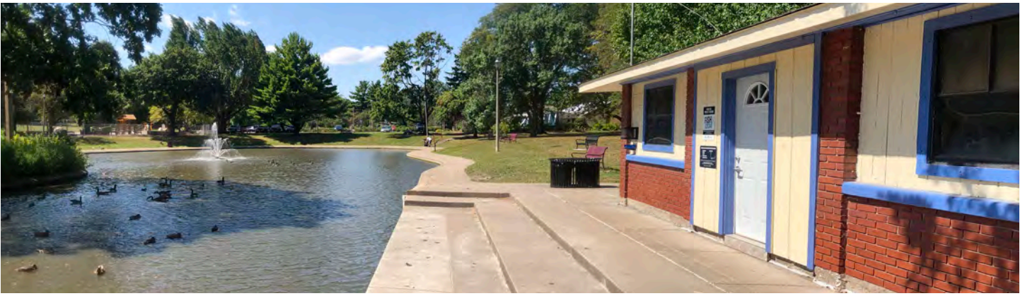
Warming House along Lagoon
