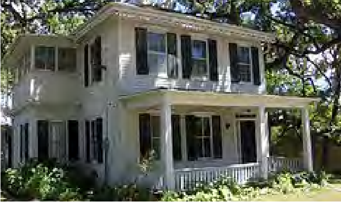
Front of Collins House
