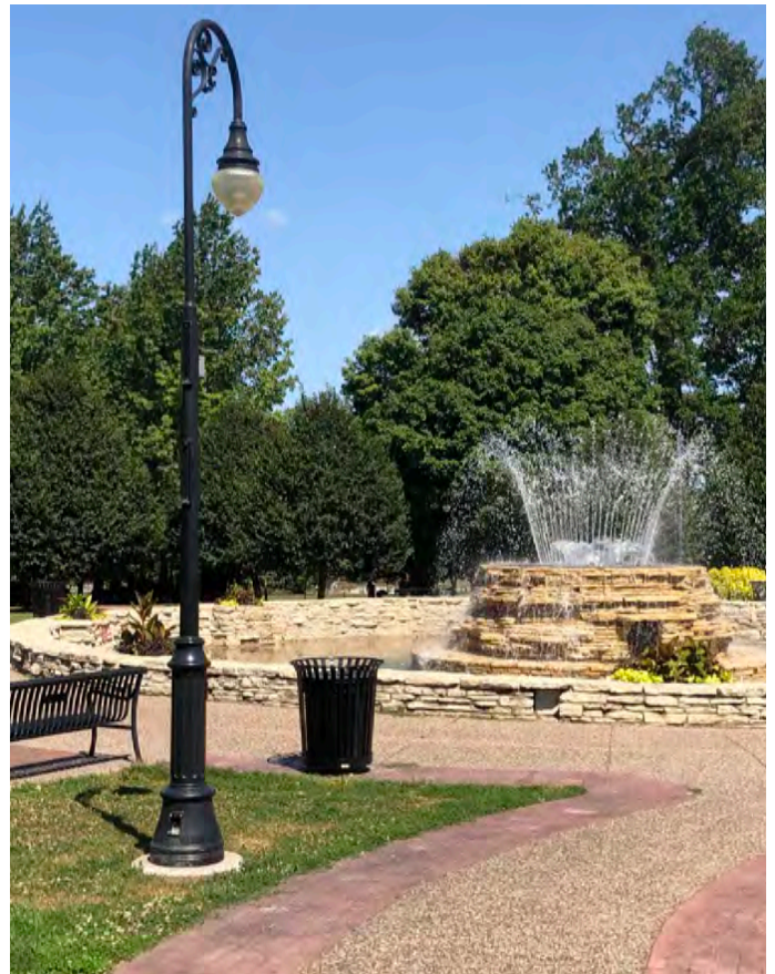
Light Pole near Fountain PARKS CONDITION ASSESSMENT
