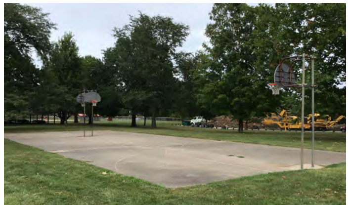
Basketball Court PARKS CONDITION ASSESSMENT
