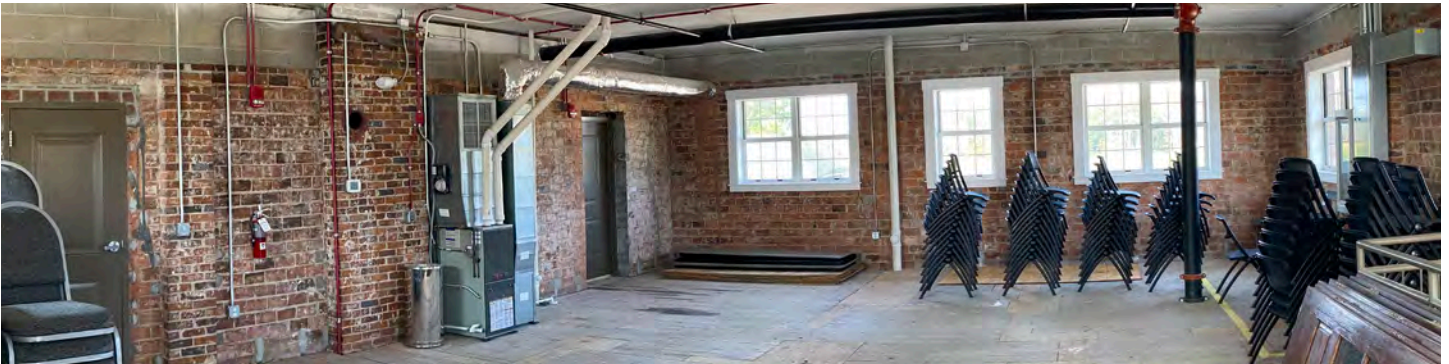
Upstairs Storage Area
