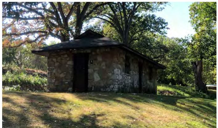
Restroom near Playground
