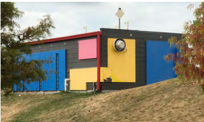
Restroom Facility at Spray Park
