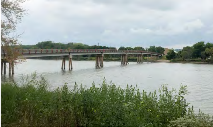
Pedestrian Bridge to S. Concord Street
