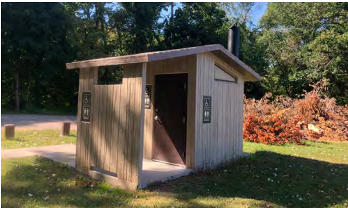
Restrooms near Bathroom
