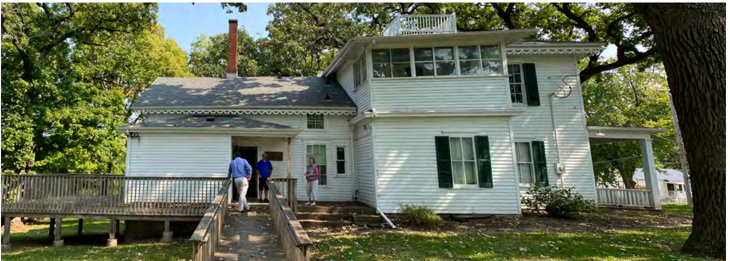
Accessible Entrance to Collins House
