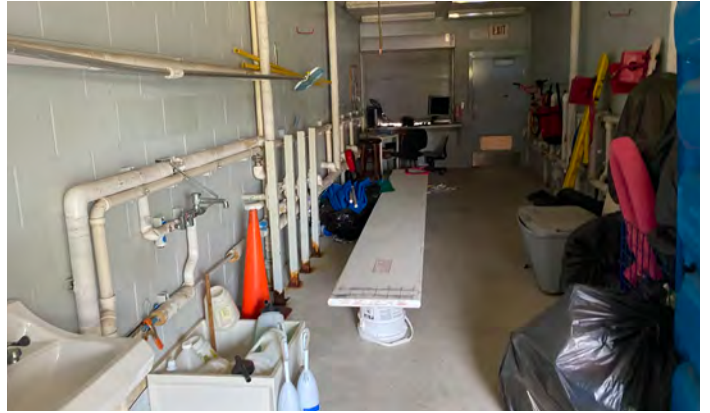
Storage and Utility Room
