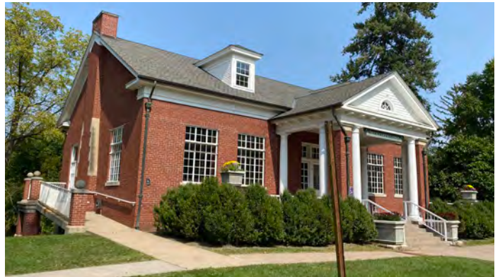
Accessible Entrance along Side
